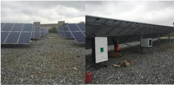
Fig. 3. a) Front view of the solar field (left). b) Back view from the solar field (right). The white box on the left is the Schneider Electric Inverter.
