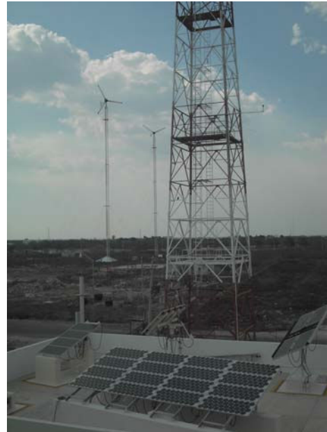
Figure 2. Photovoltaics modules in the FI-UADY
